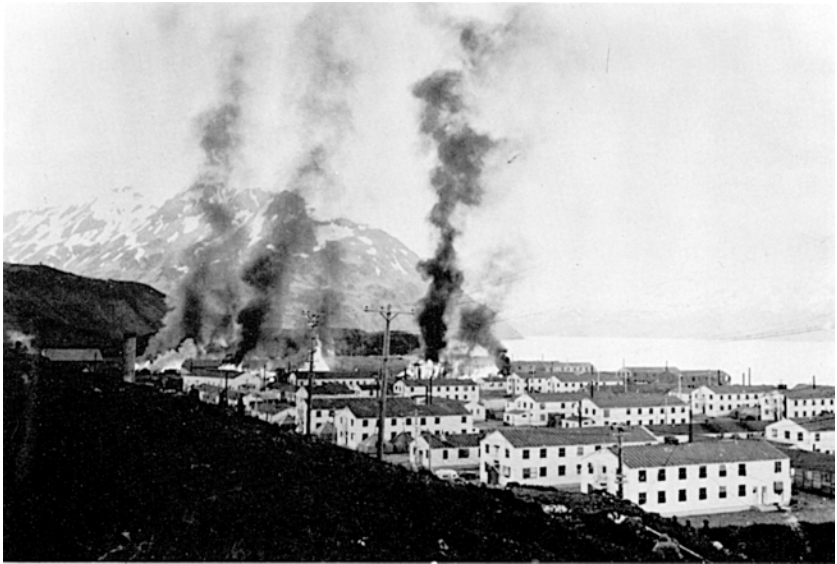
Buildings burning after the first enemy attack on Dutch Harbor, 3 June 1942. (DA photograph)
